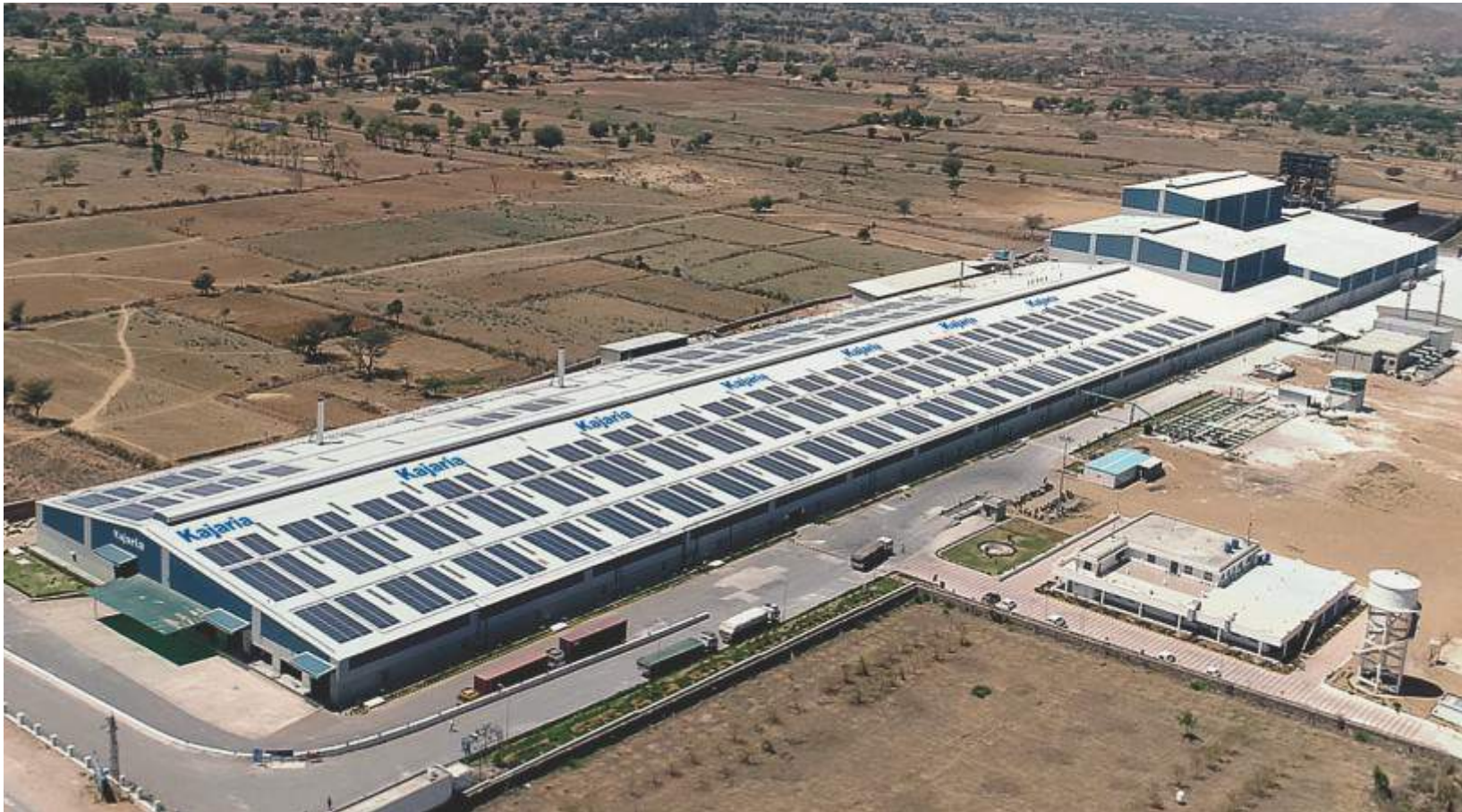
Aerial view of Virat Nagar Plant (Rajasthan)
